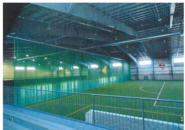
Arched “STEELWAY” structure (St-Eustache multisport complex – TX-38)
