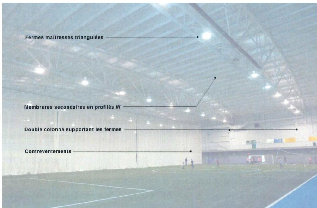
Fig. 32 – Overall view of the Artopex Complex with comparison of similar structural elements (ABCP infographic)
