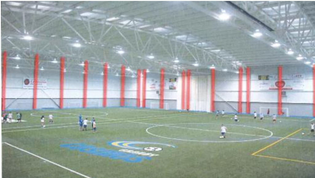
Fig. 17 – Steel columns on the periphery of the building (ABCP infographic on a photograph representing the Artopex Complex)
