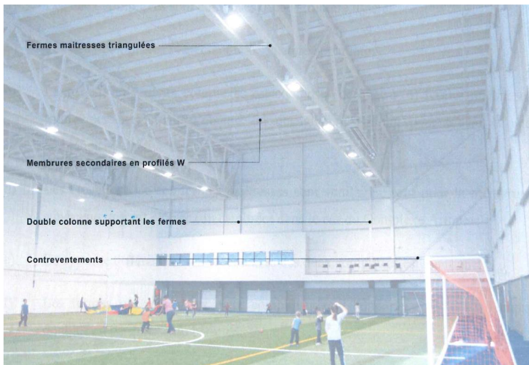
Fig. 33 – Overall view of the Victoriaville Complex with comparison of similar structural elements (ABCP infographic)
