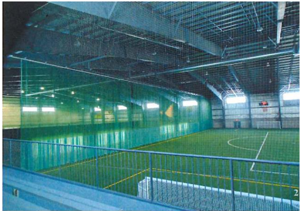
Arched “STEELWAY” structure (St-Eustache multisport complex –TX-38)
