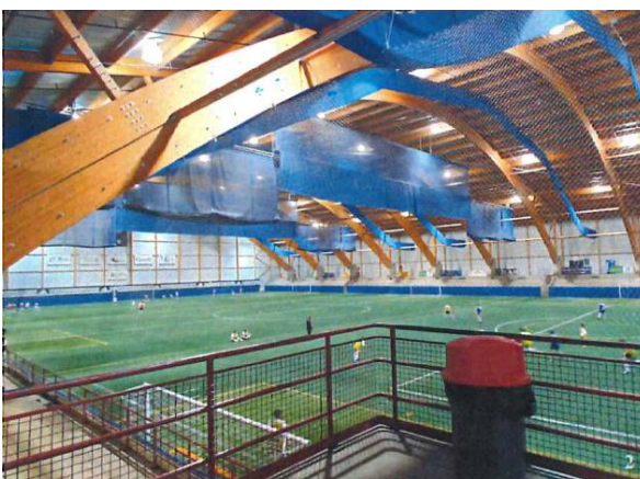
Wood structure (Laval multisport complex – TX-37)
