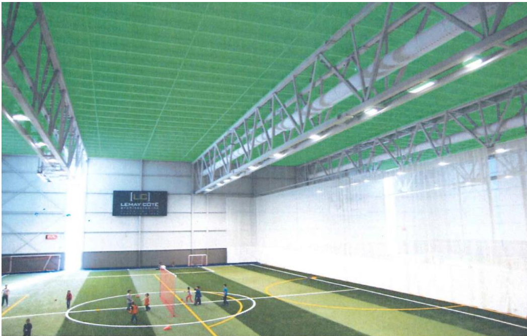
Fig. 23 – Secondary chords fixed to the cantilever chords and roof bridging (ABCP infographic on a photograph representing the Victoriaville Complex)
