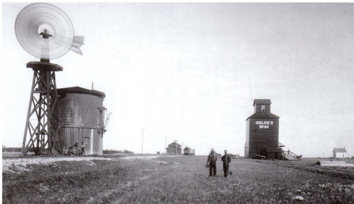
A typical Prairie windmill-powered water pump and adjacent locomotive fuel water tower, with the freight and passenger station way beyond, and a private grain elevator on CPR land.
