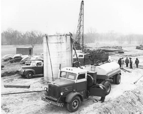
As shown in this historic photograph, the first hydraulic fracture treatment was performed by Halliburton under license to Stanolind Oil Company on March 17, 1949, east of Duncan, Ok. Hydraulic fracturing has since allowed commercial hydrocarbon recovery from more than 1 million wells that could not have produced economically, and that number grows by the day with nearly every U.S. gas well and the majority of all U.S. oil wells now being hydraulically fractured.
